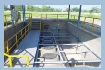
**Figure 3.10** Johkasou system for treating wastewater from Ruk Singwadlom dormitory
