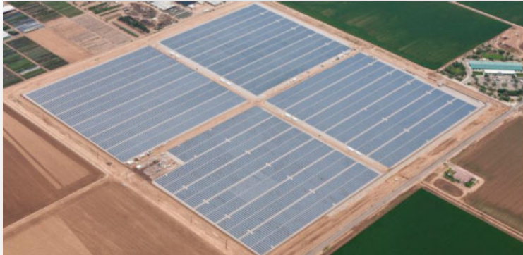
Arizona in USA, single axis tracker (25 MW)
