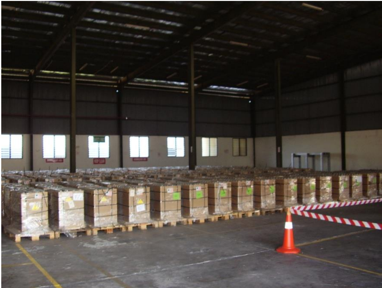
Spacious area with high roof and air ventilation
