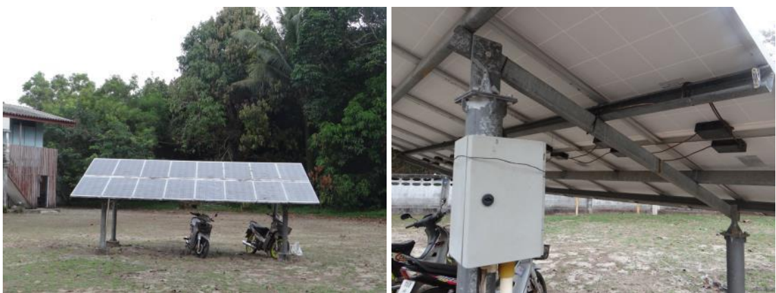
Figure 15: 2 kW p PV system powering the public health centre
