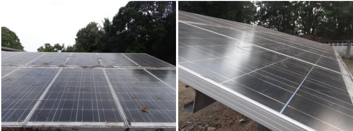
Figure 16: Dirty crystalline solar modules
