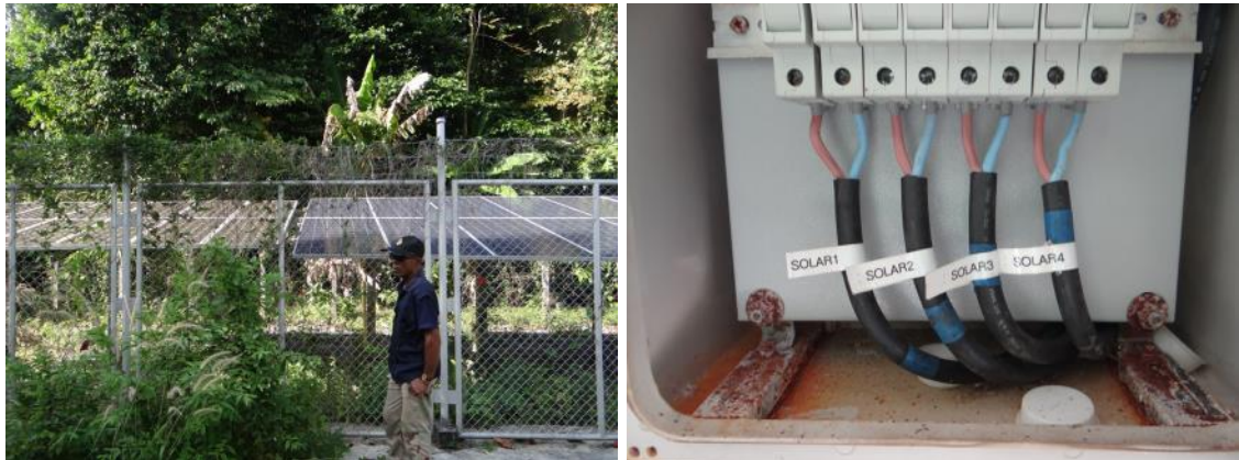
Figure 21: PV system supplying the electricity for the BTS1 (PV1) and rusty components
