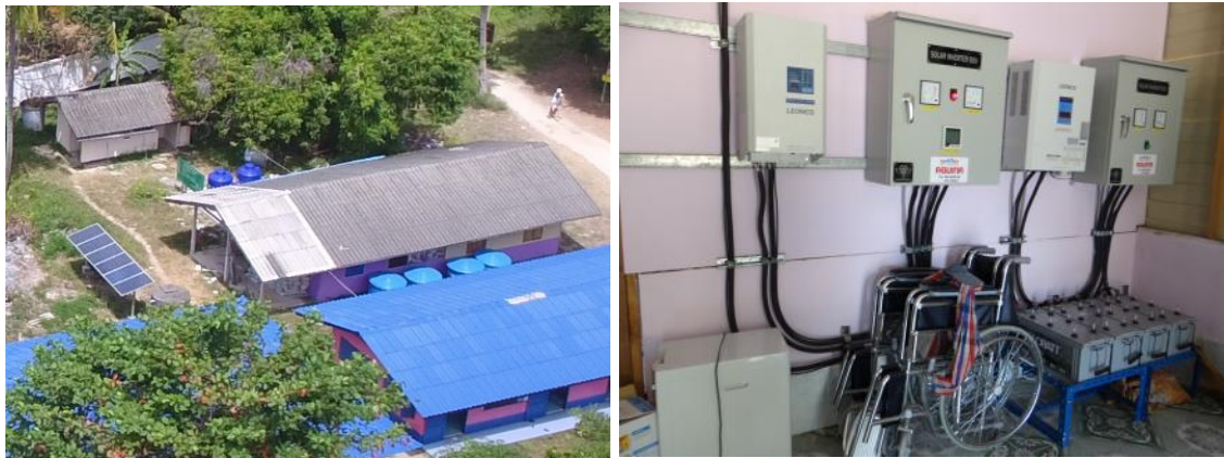
Figure 17: PV-battery system supplying public health centre
