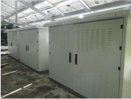
Figure 24: Battery cabinets
