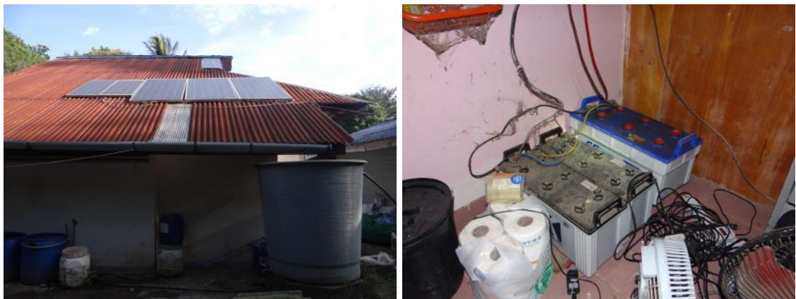
Figure 12: Solar Home System with batteries
