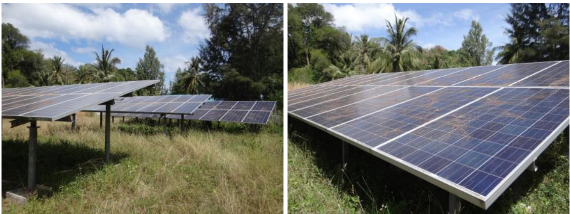
Figure 15: Dirty PV modules observed
