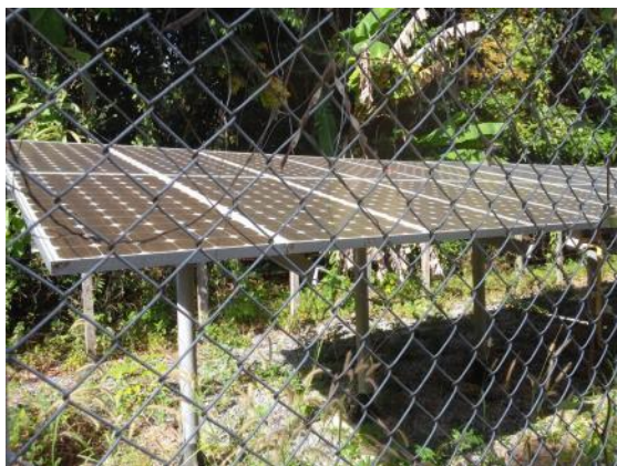
Figure 42: Twelve broken SHARP modules at BTS1
