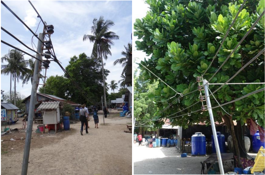
Figure 33: Steel pole of main grid
