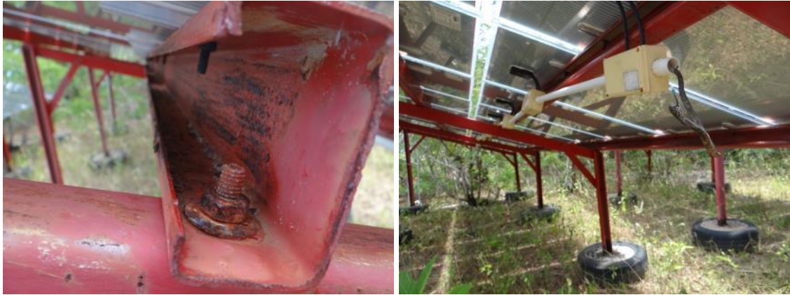
Figure 16: Rusty metal [left] and disconnected cable [right]
