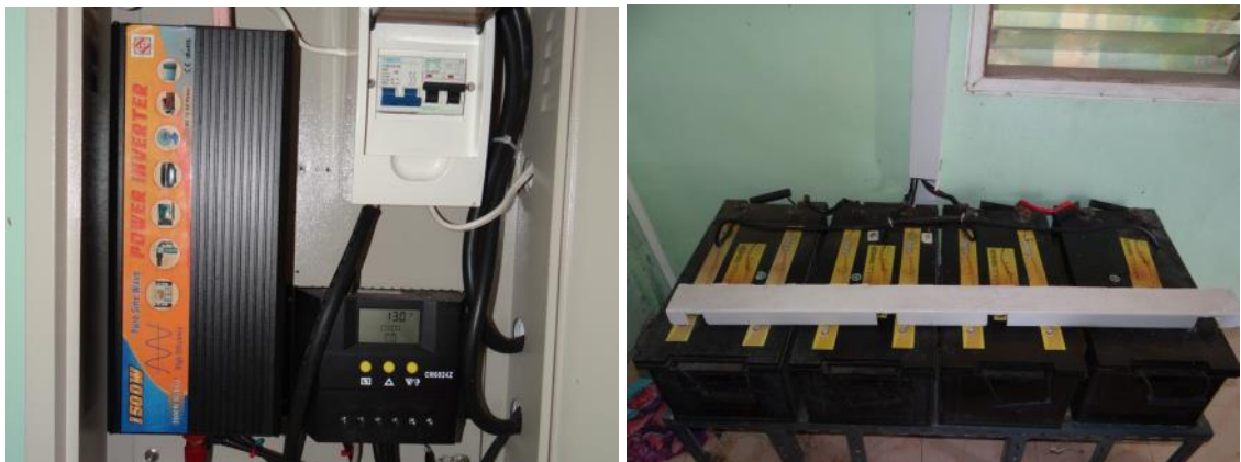
Figure 22: Inverter and charge controller [left], four Globatt batteries [right]
