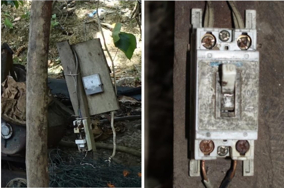
Figure 35: Disconnect Switch and Circuit Breaker for Generators
