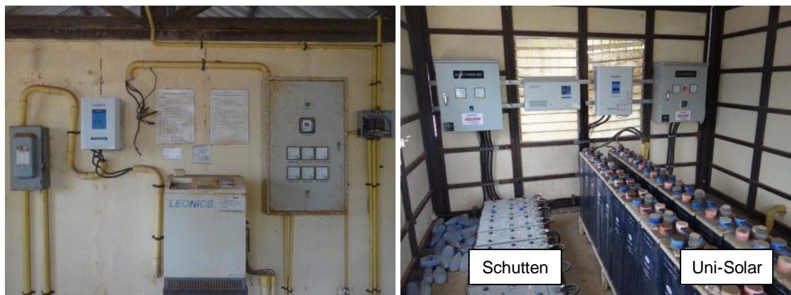
Figure 18: Inverter and batteries system inside powerhouse
