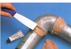
Fixing leaky pipes
